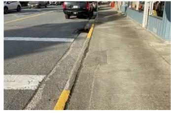
Photo 4 - Pedestrian Ramp lacking detectable warning mat and flat landing
