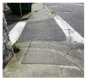
Photo 5 – Pedestrian Curb Ramp lacking detectable warning mat
